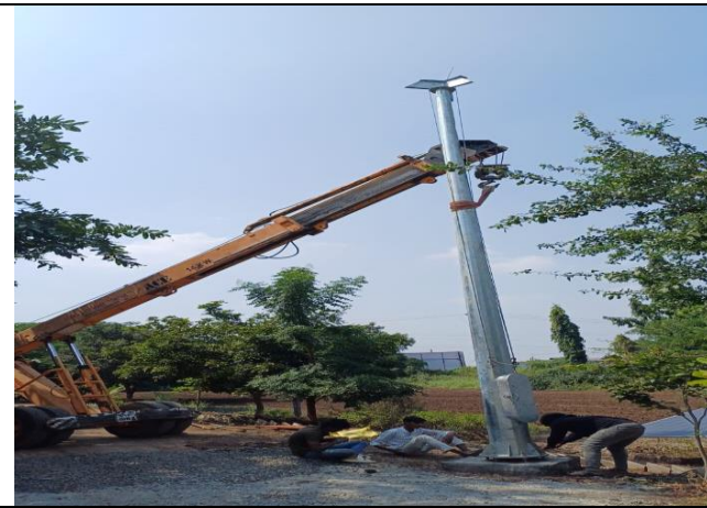
Installation of Solar High Mast at POCRTC, Pandharpur
