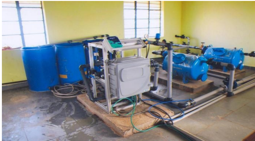
Automatic fertigation installed at PGI farm, MPKV, Rahuri
